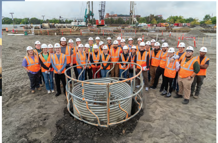
CEE students tour the construction site during caisson installation.
